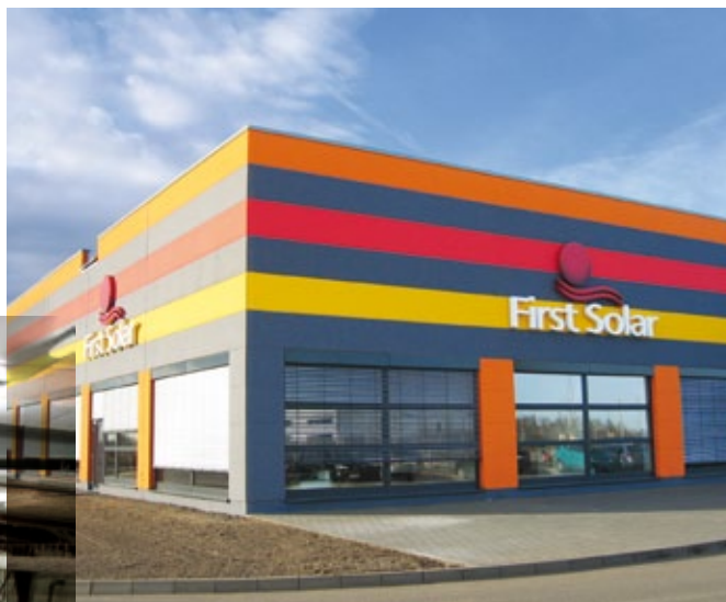
First Solar's Manufacture Research and Design Campus —
